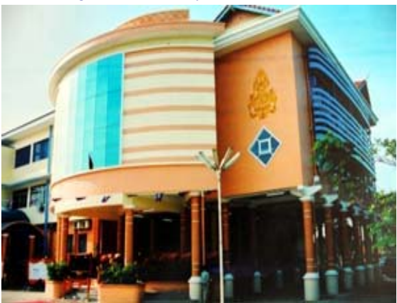
A new building at the Royal University of Law And economy in Phnom Penh
