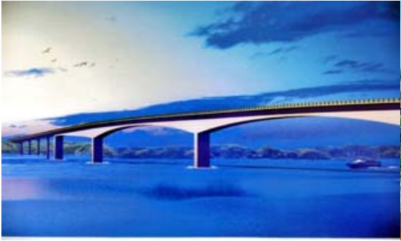
Se Kong Bridge in Stung Treng province
