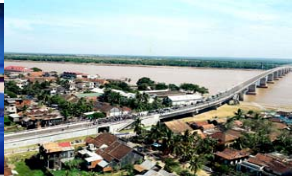
Kizona Bridge in Kampong Cham province
